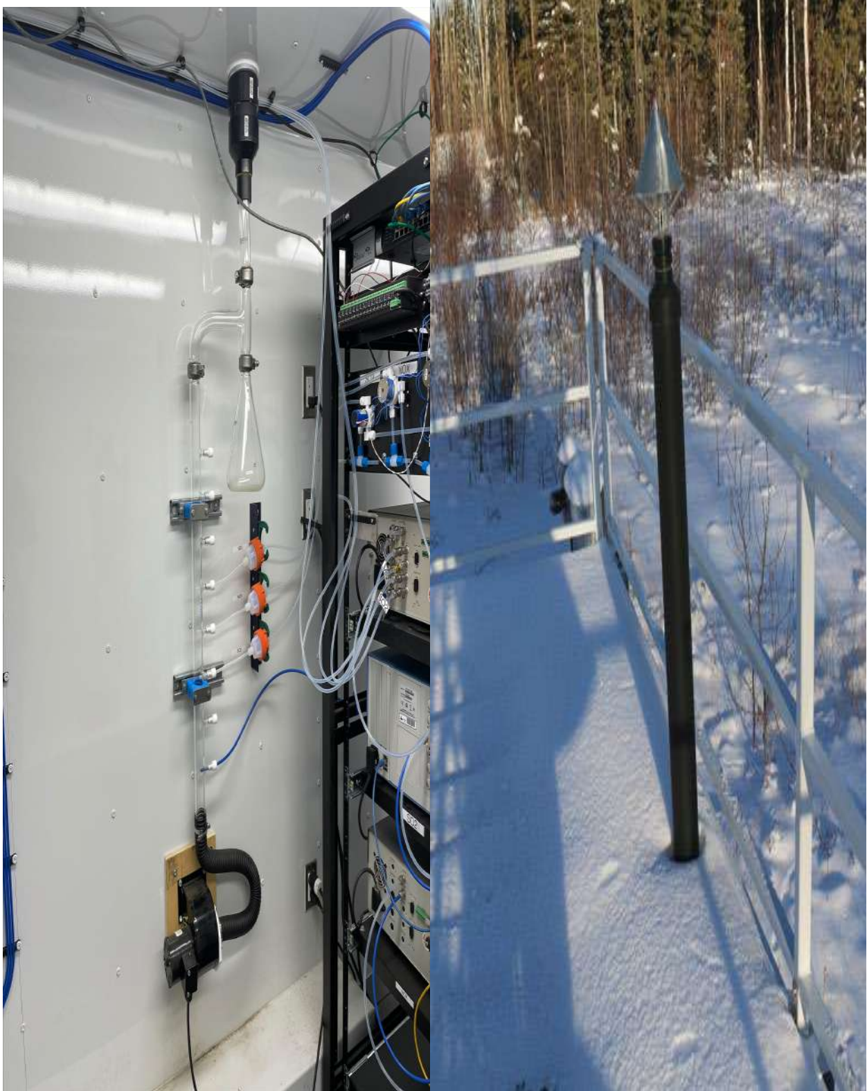
Figure 10 – Photo showing the inlet and sample manifold.
