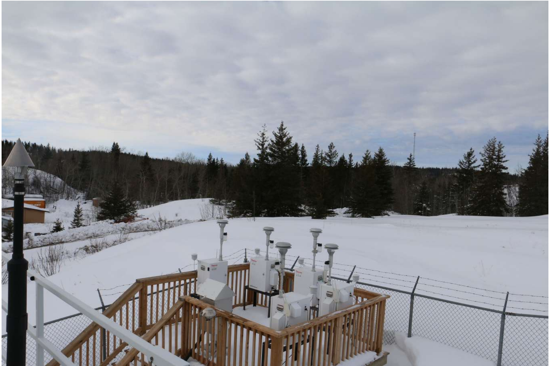
Figure 6.3 – Environment looking West
