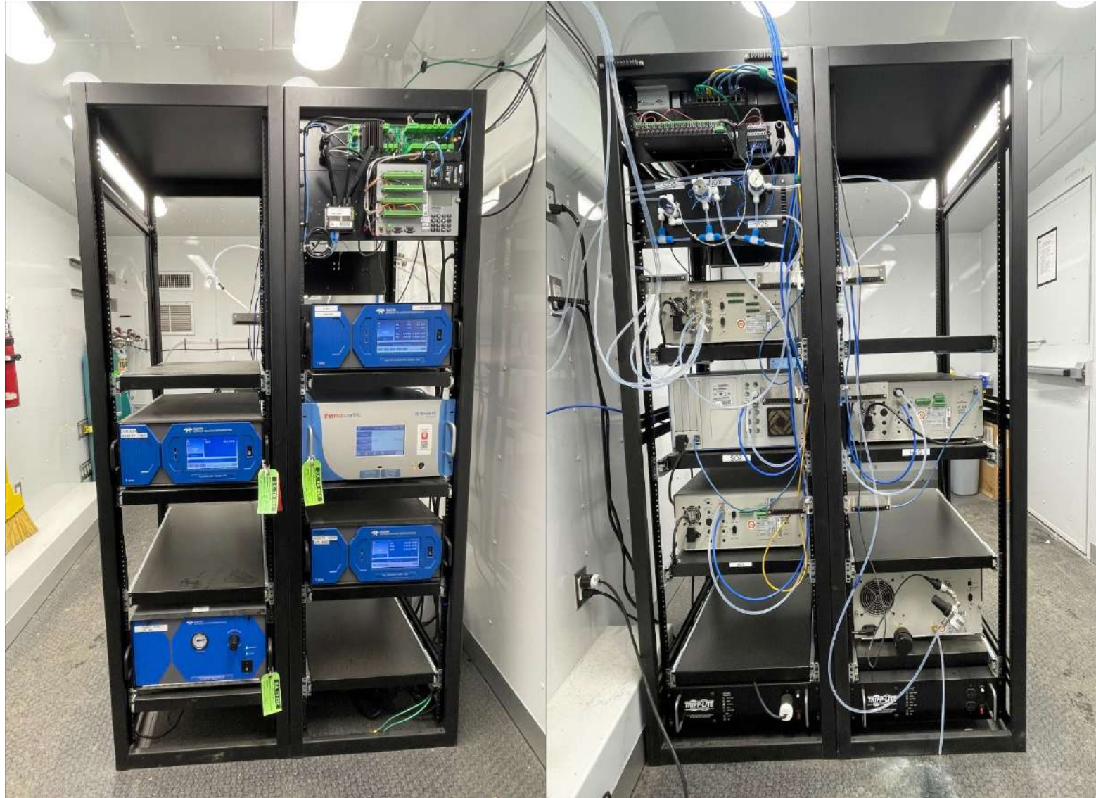
Figure 12 –Photo of the front and the back of instrument rack
