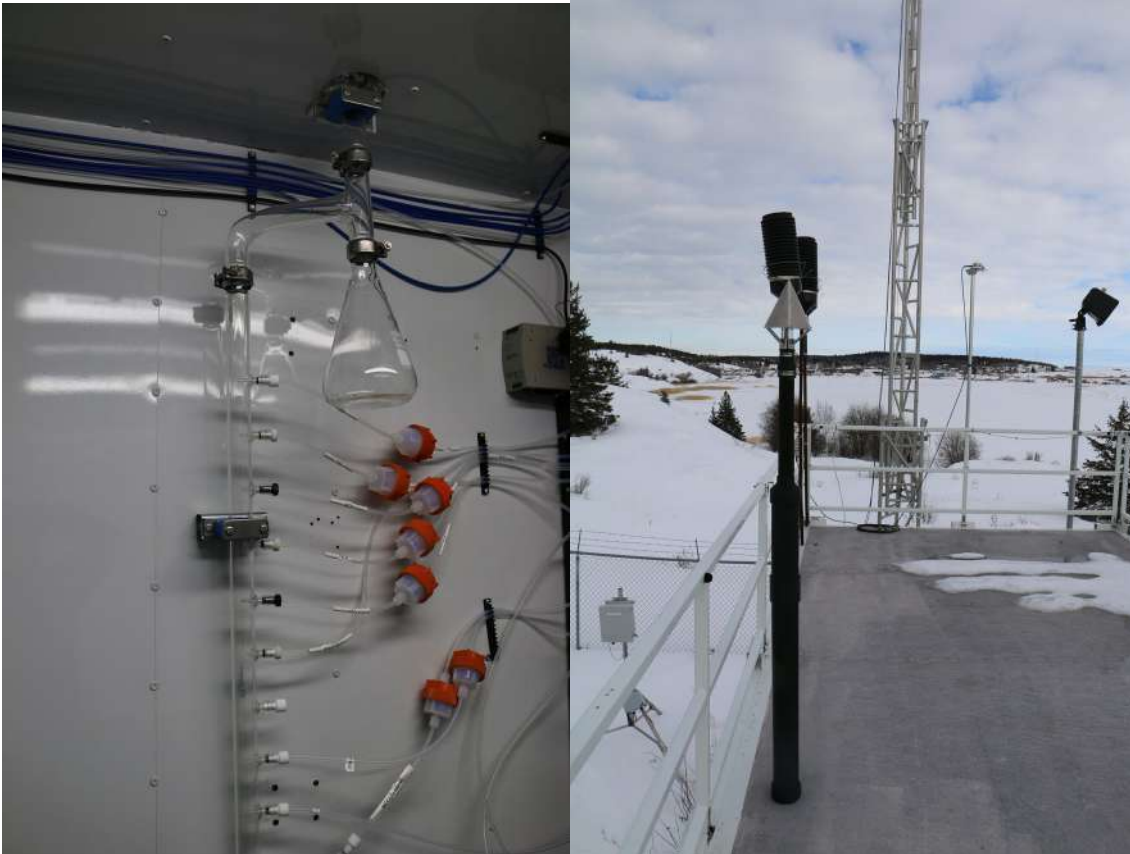
Figure 7.0 – Photo showing the inlet and sample manifold
