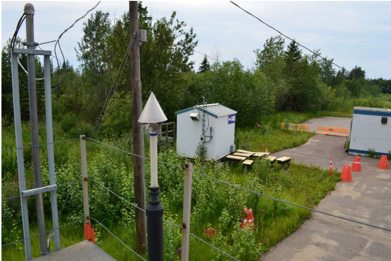
Figure 6.3 – Environment looking West
