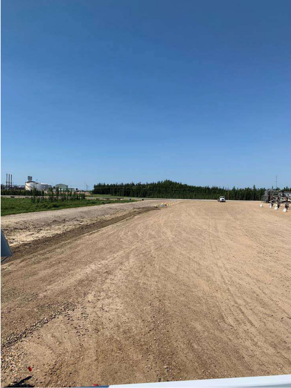
Figure 8 – Environment looking West
