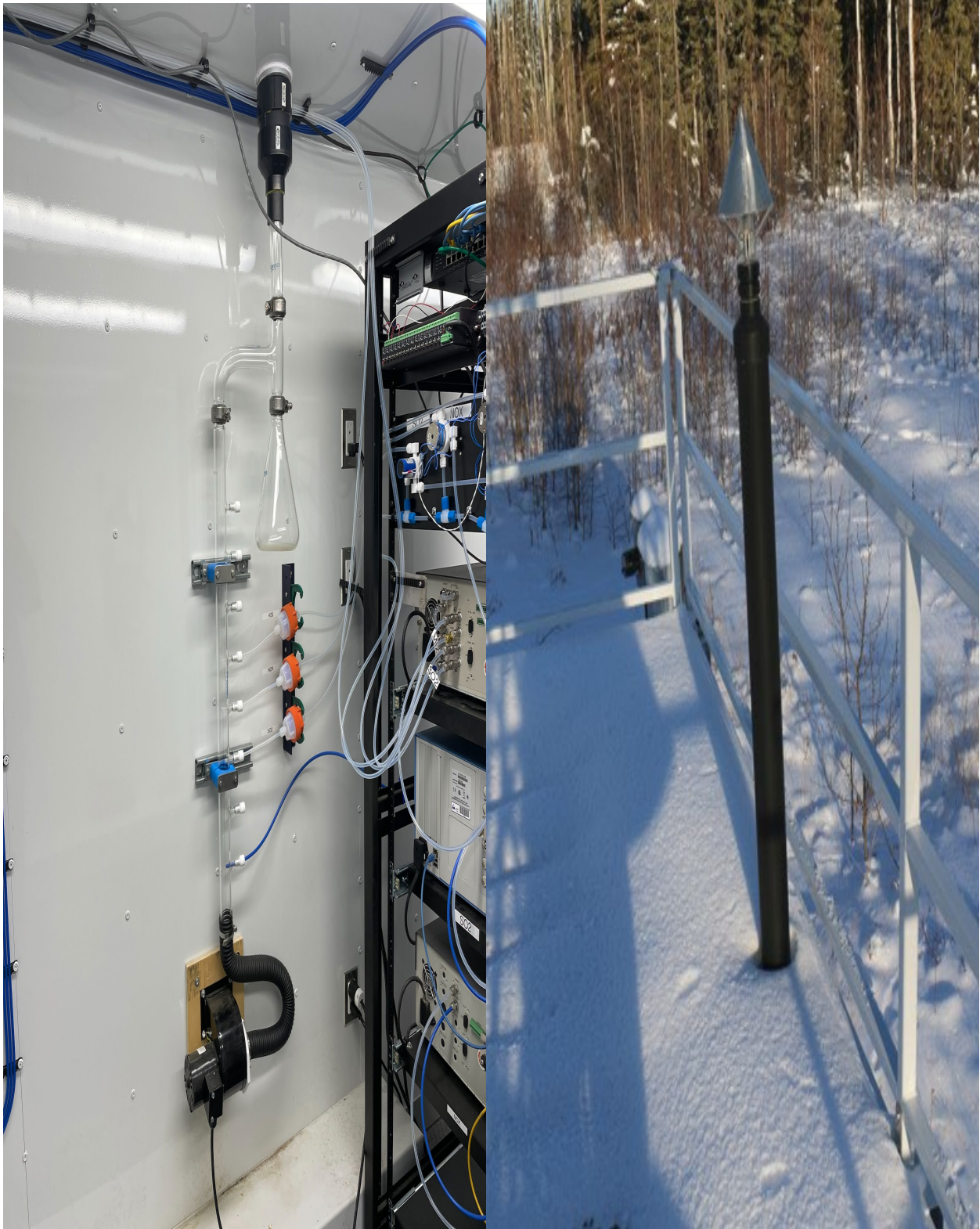
Figure 9 – Photo showing the inlet and sample manifold.
