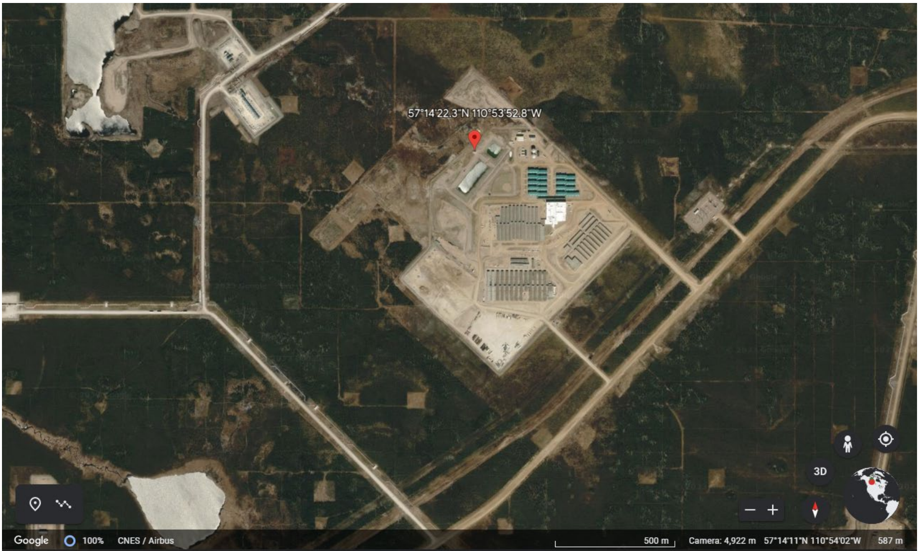
Figure 3 – Aerial photo showing AMS 19 - Firebag
