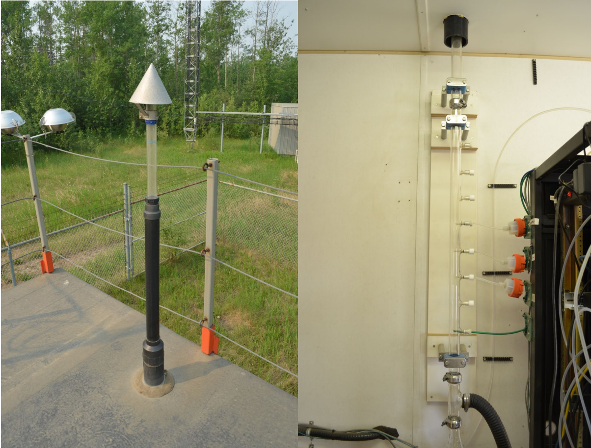
Figure 10 – Photo showing the inlet and sample manifold
