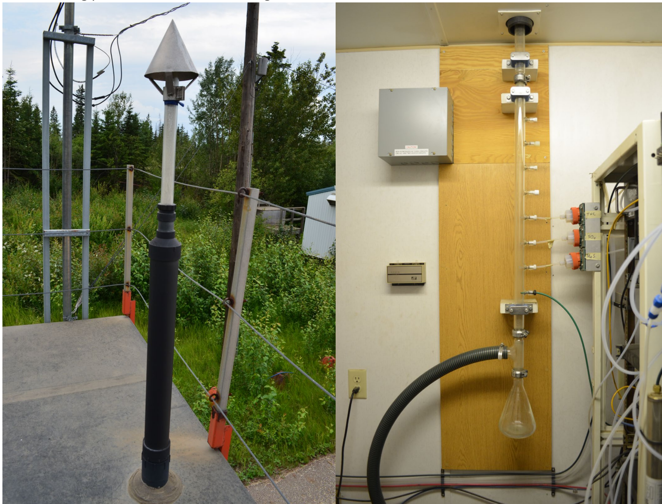
Figure 10 – Photo showing the inlet and sample manifold
