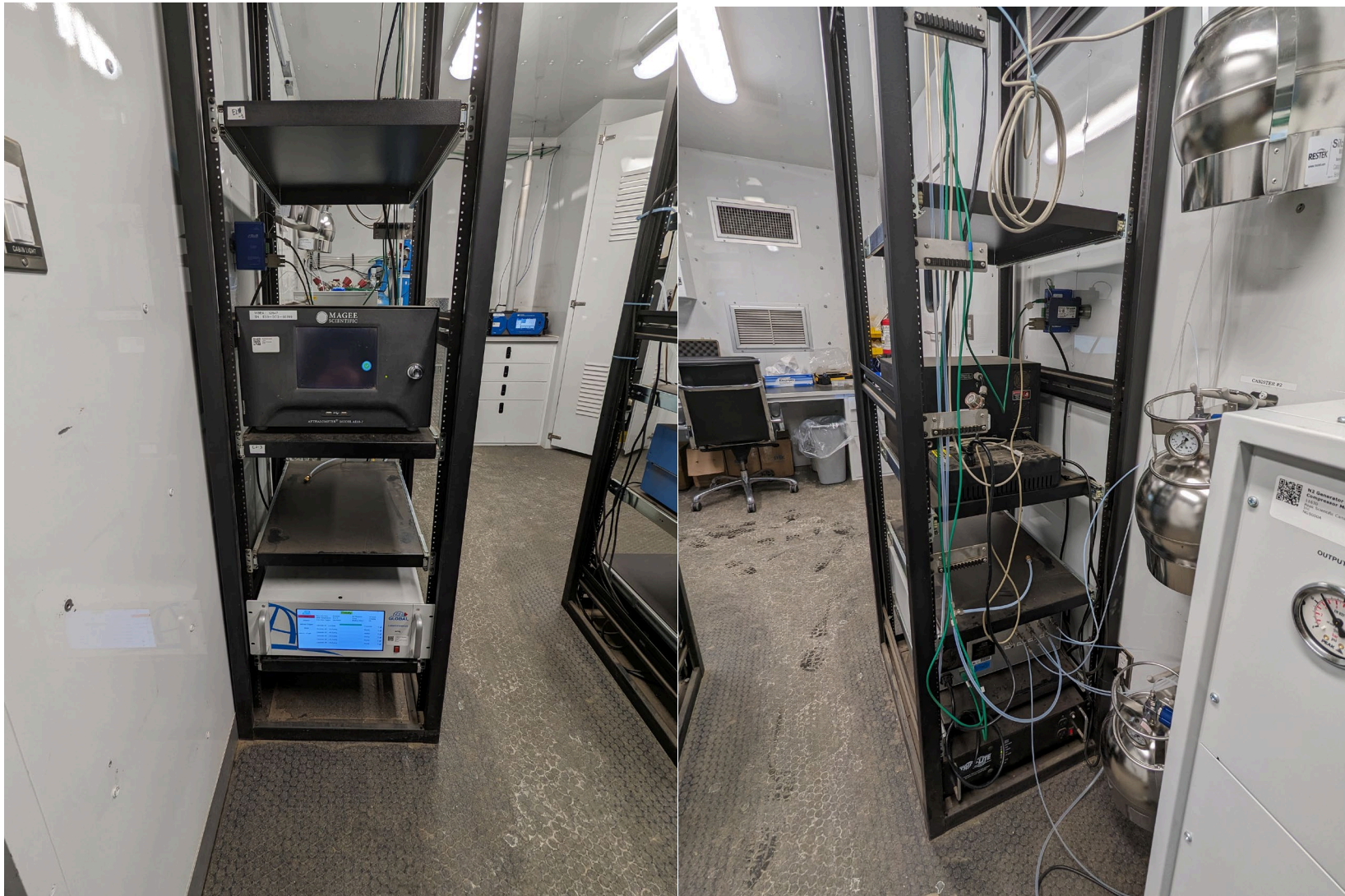
Figure 13 –Photo of the front and the back of the instrument rack
