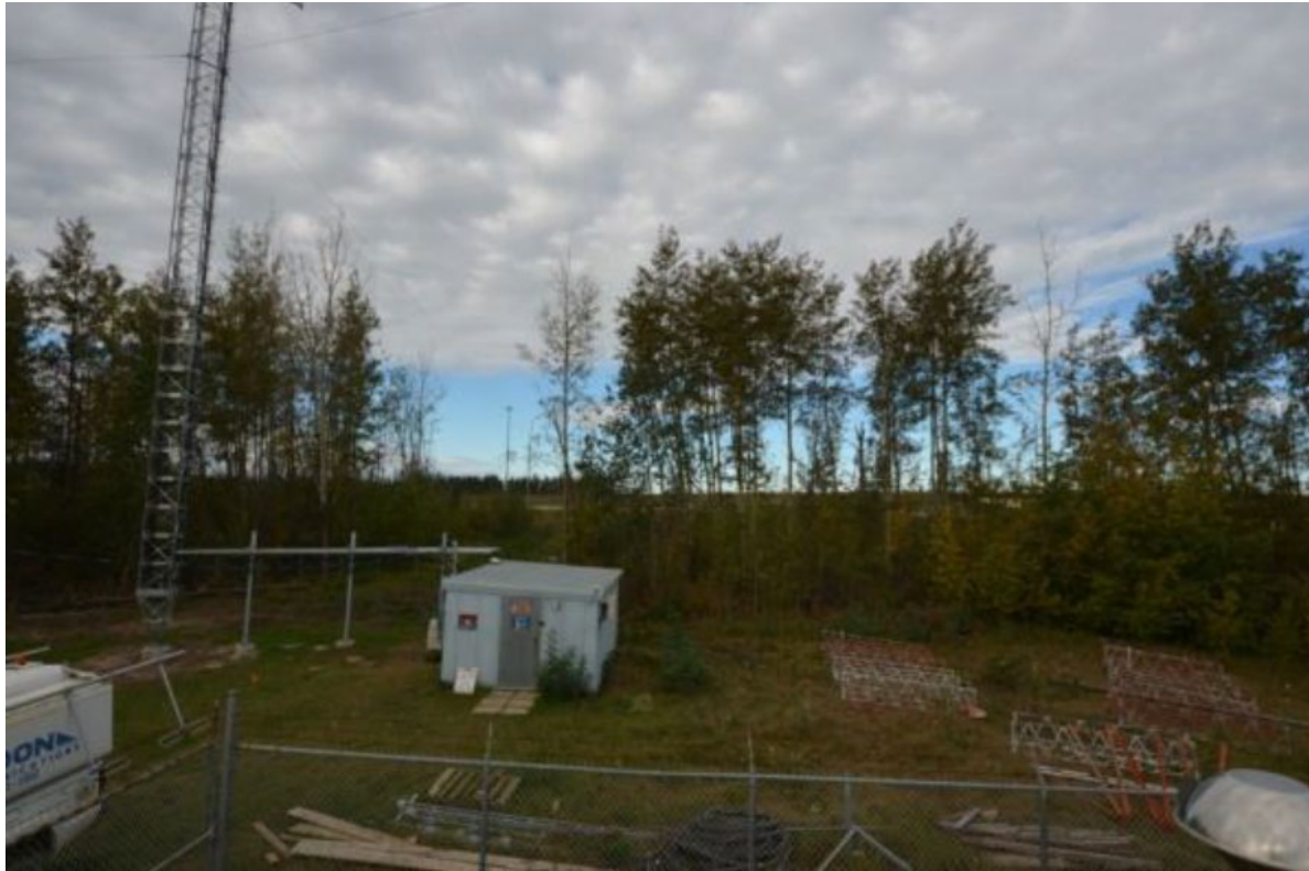
Figure 6.3 – Environment looking West
