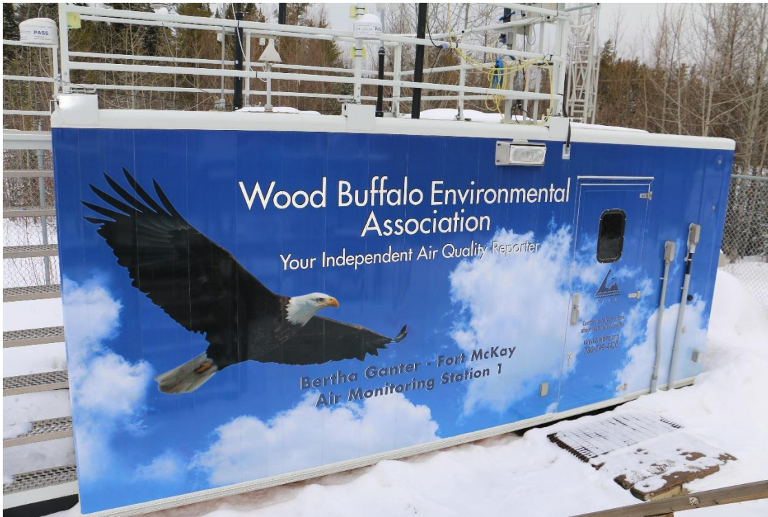
Figure 4.0 – Exterior of monitoring station
