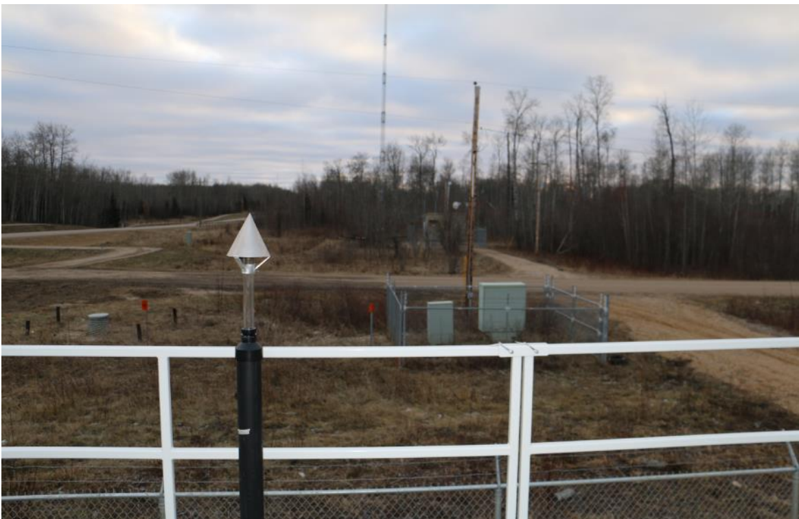
Figure 4.3 – Environ looking south
