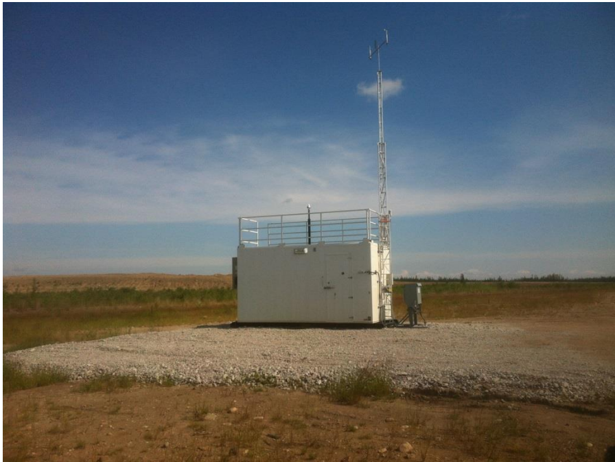
Figure 4.0 – Exterior of monitoring station
