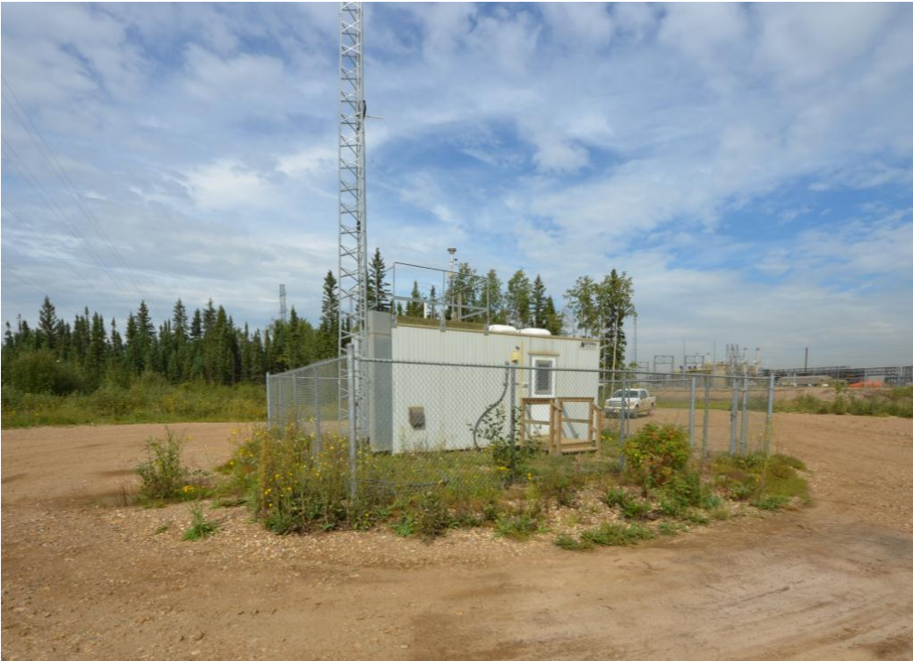
Figure 4.0 – Exterior of monitoring station looking north
