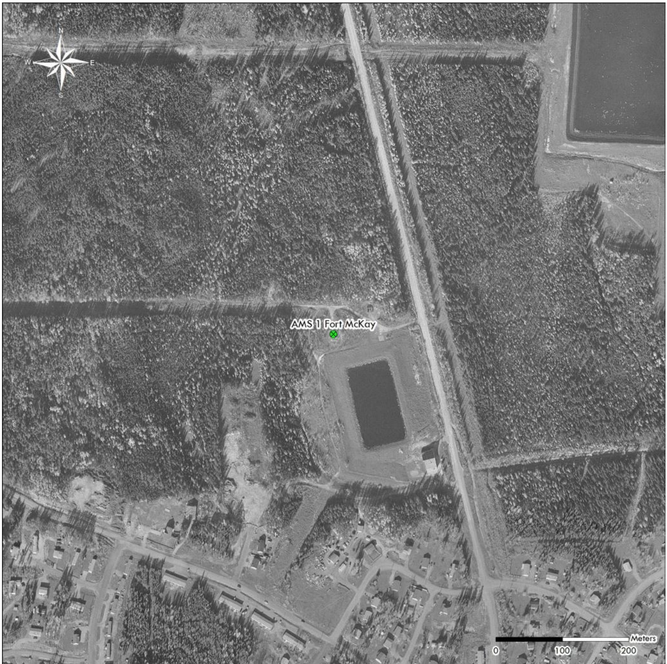
Figure 3.0 – Aerial photo showing AMS 01 – Fort McKay - Bertha Ganter Station
