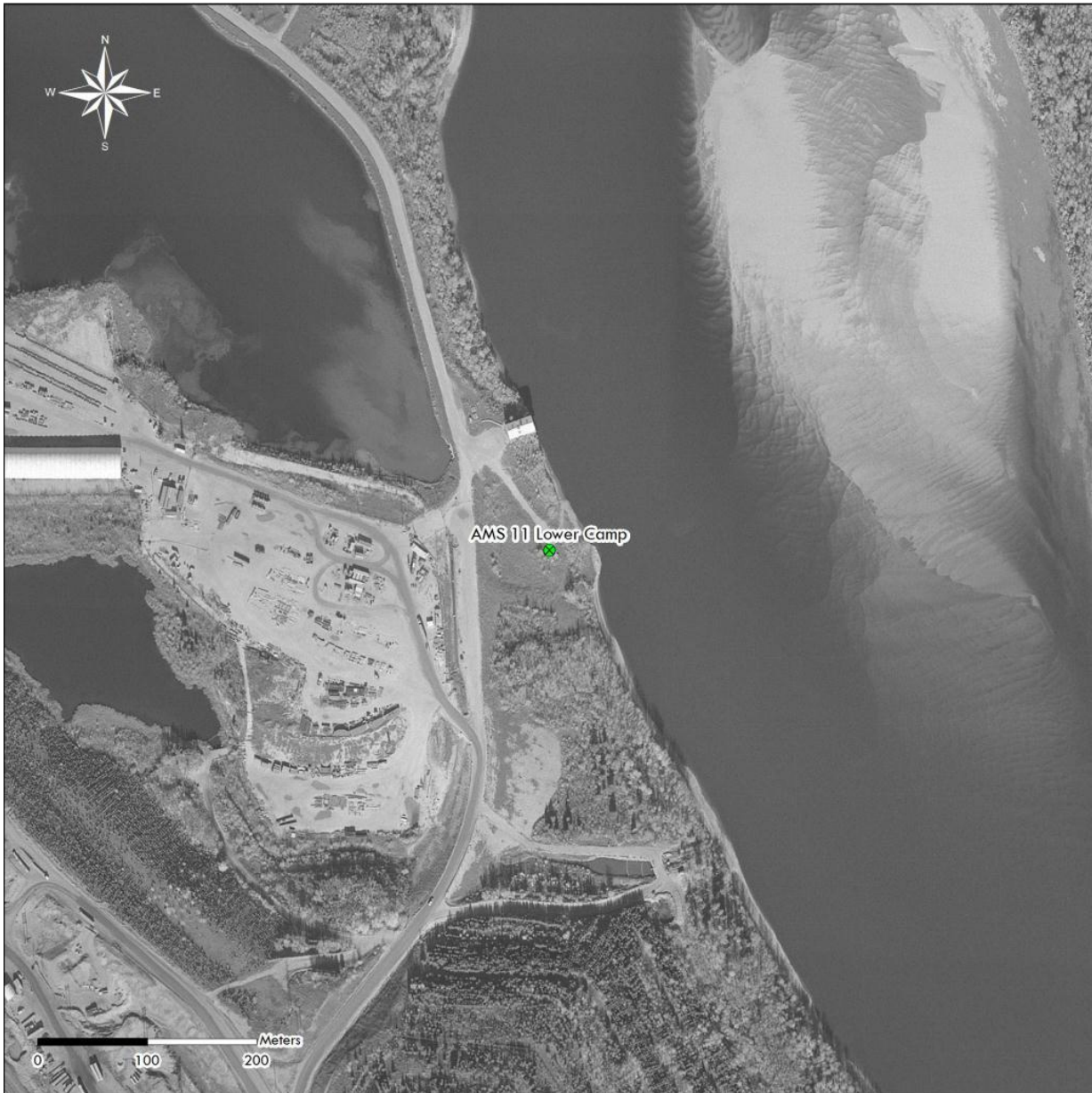
Figure 3.0 – Aerial photo showing AMS 11 – Lower Camp Station
