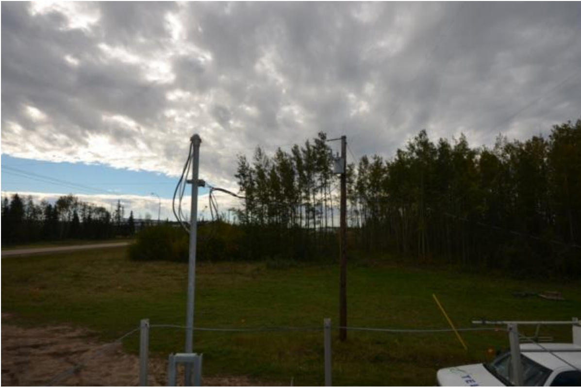
Figure 4.4 – Environ looking south
