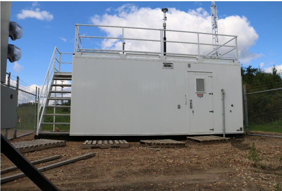
Figure 4.1 – Exterior of AMS 21 looking east
