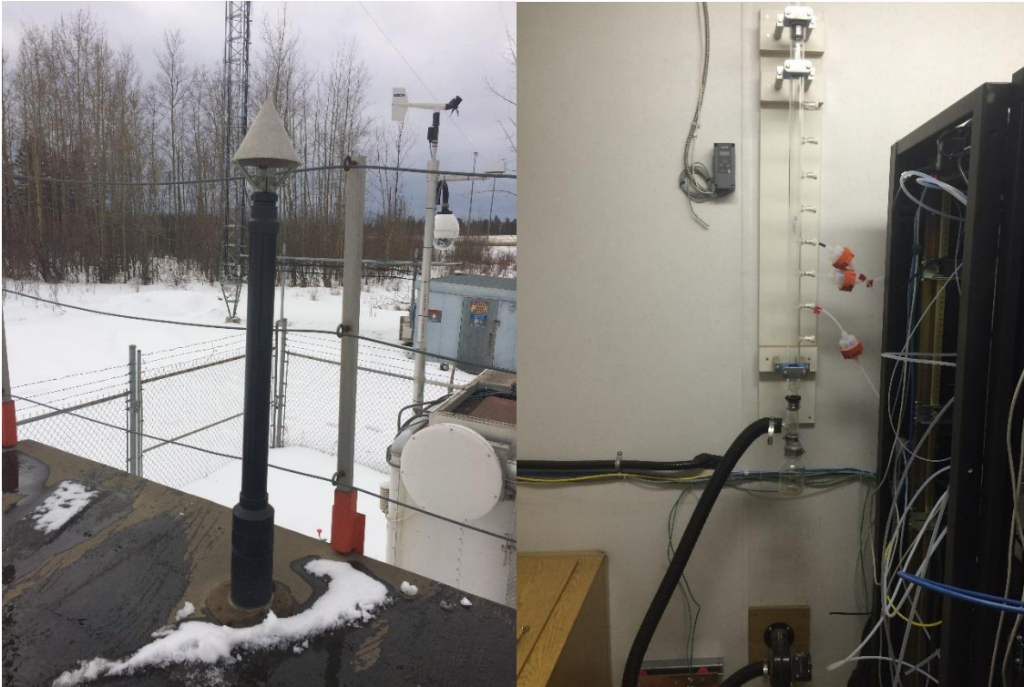
Figure 4.6 – Outdoor Sample Inlet & Indoor Sample Manifold
