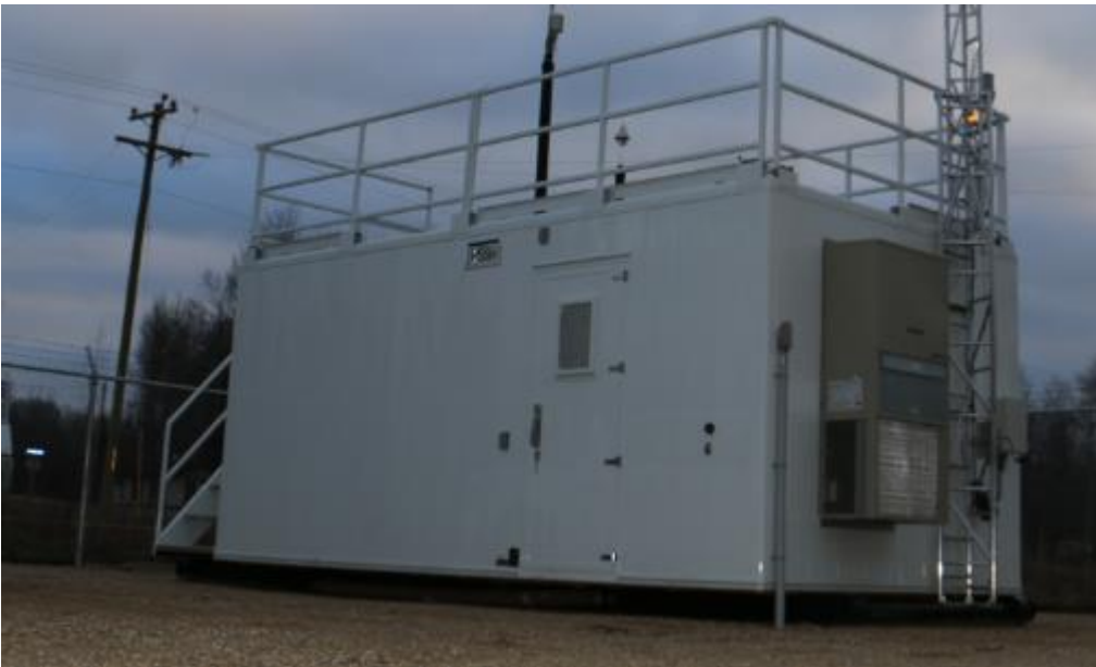
Figure 4.1 – Exterior of AMS 22 looking north
