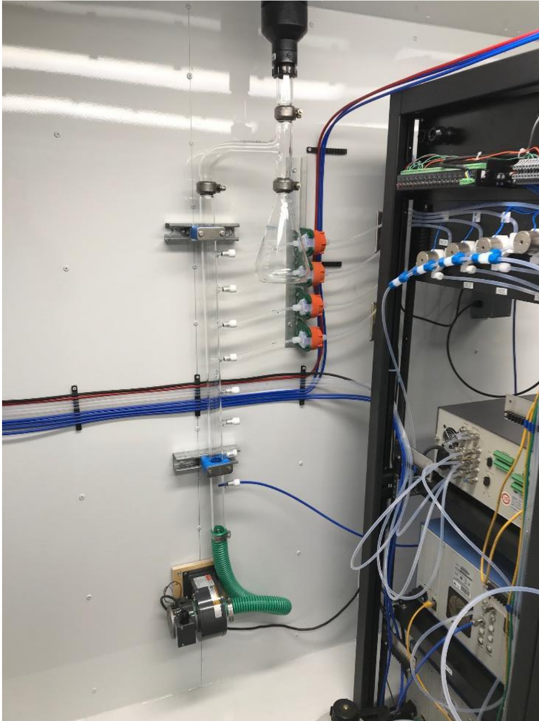
Figure 6.0 – Photo showing the inlet and sample manifold
