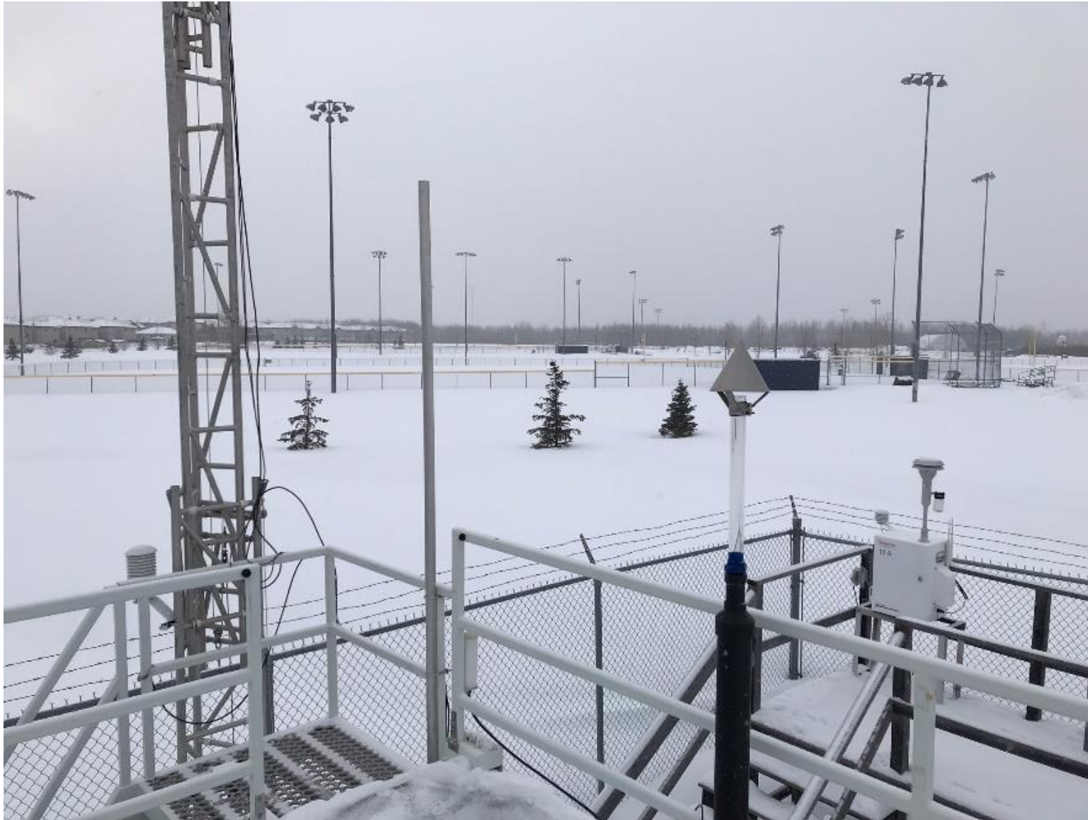
Figure 6.3 – Environment looking West
