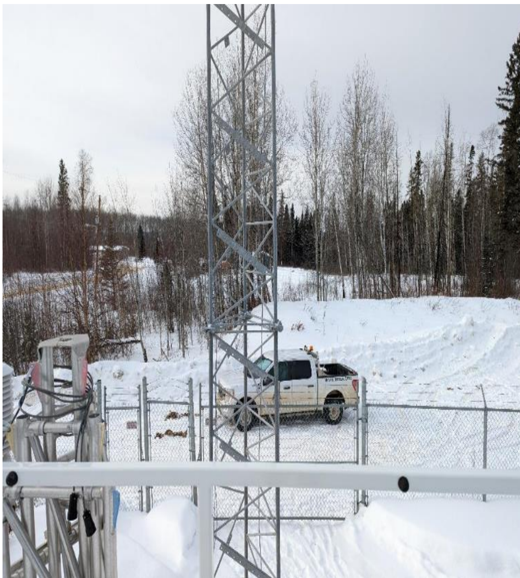
Figure 6.3 – Environment looking West
