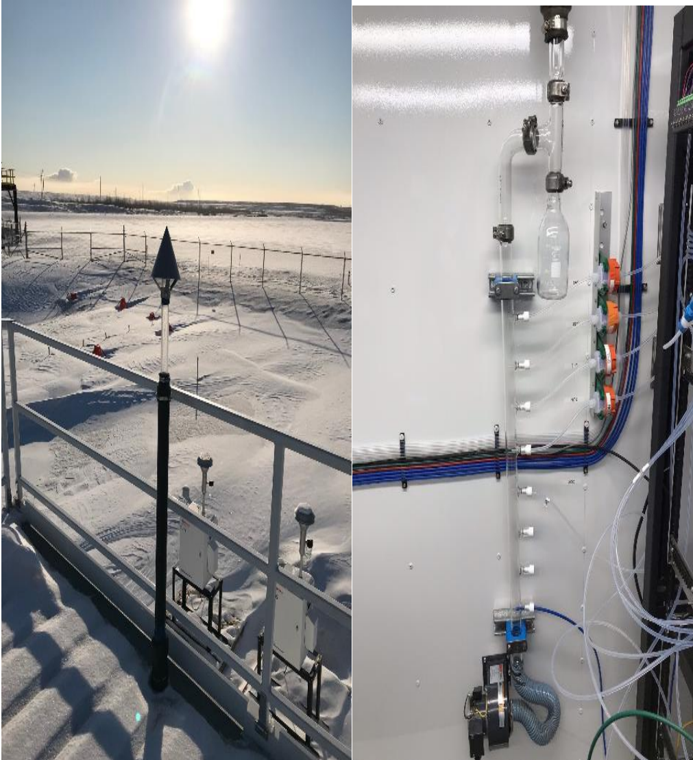
Figure 6.0 – Photo showing the inlet and sample manifold
