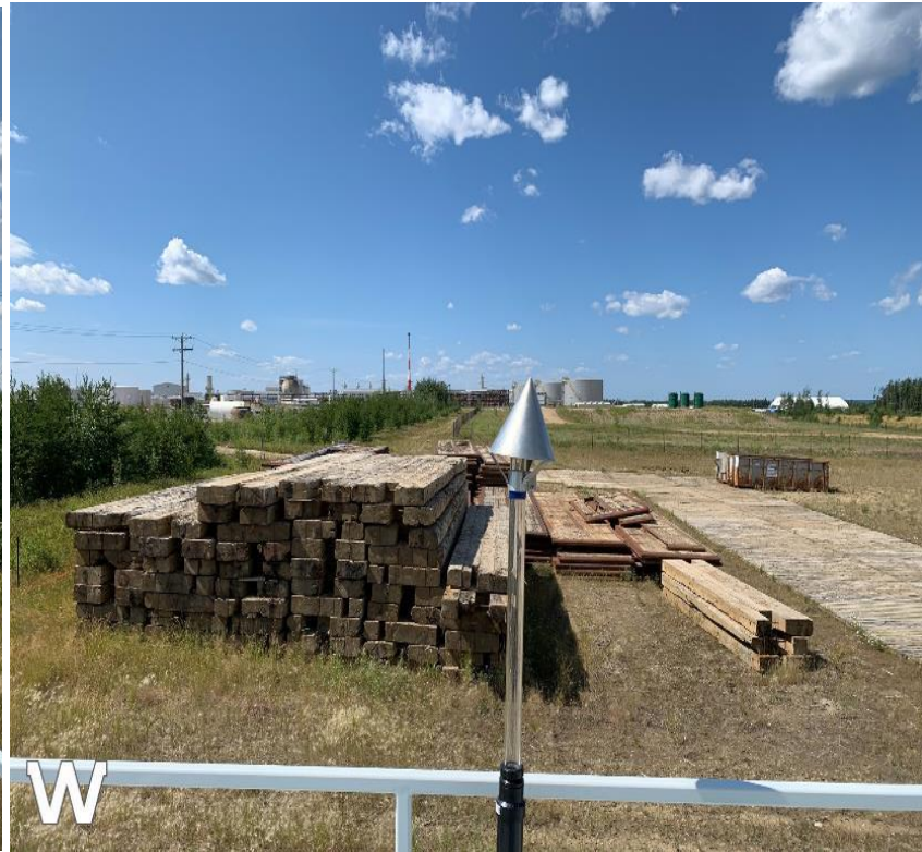
Figure 5.3 – Environment looking West
