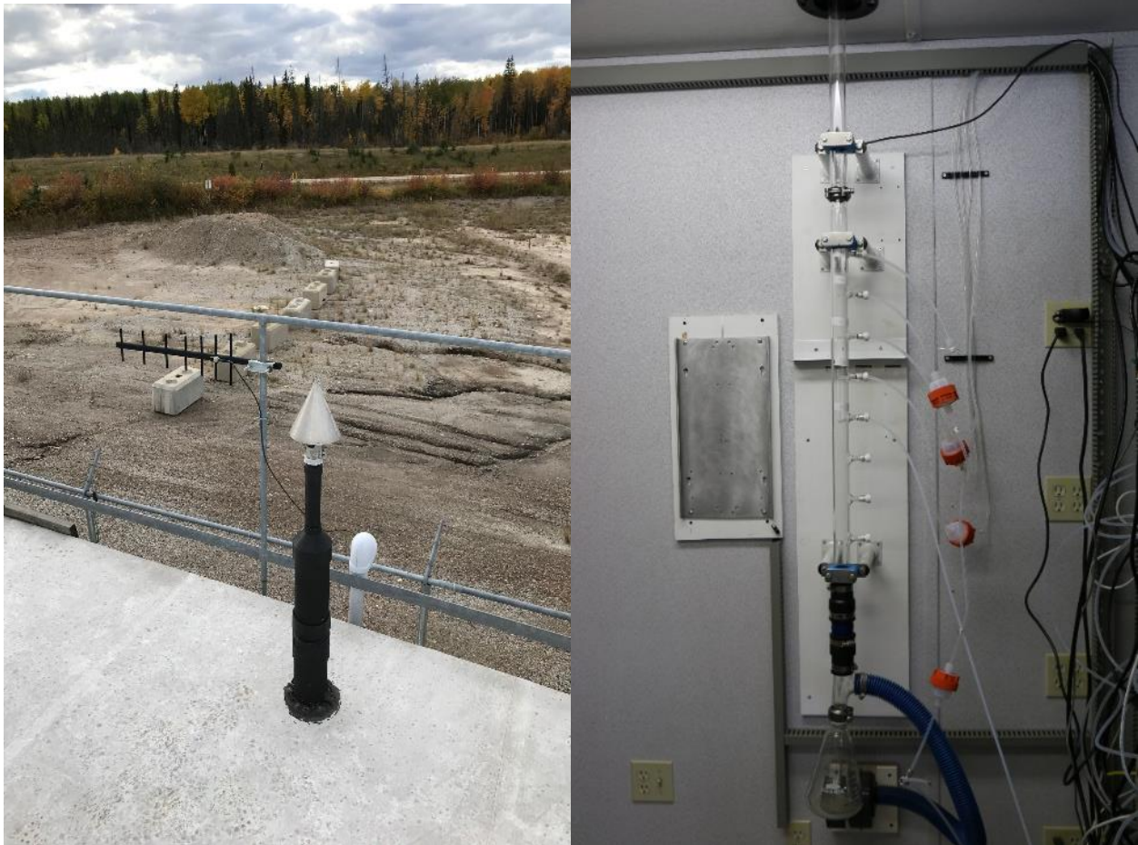
Figure 6.0 – Photo showing the inlet and sample manifold
