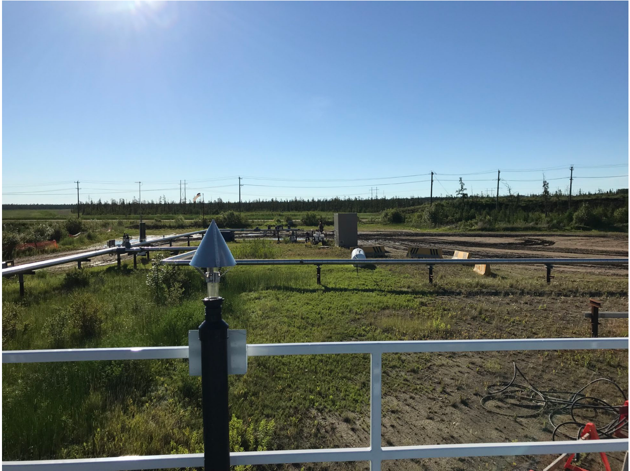
Figure 5.1 – Environ Looking East
