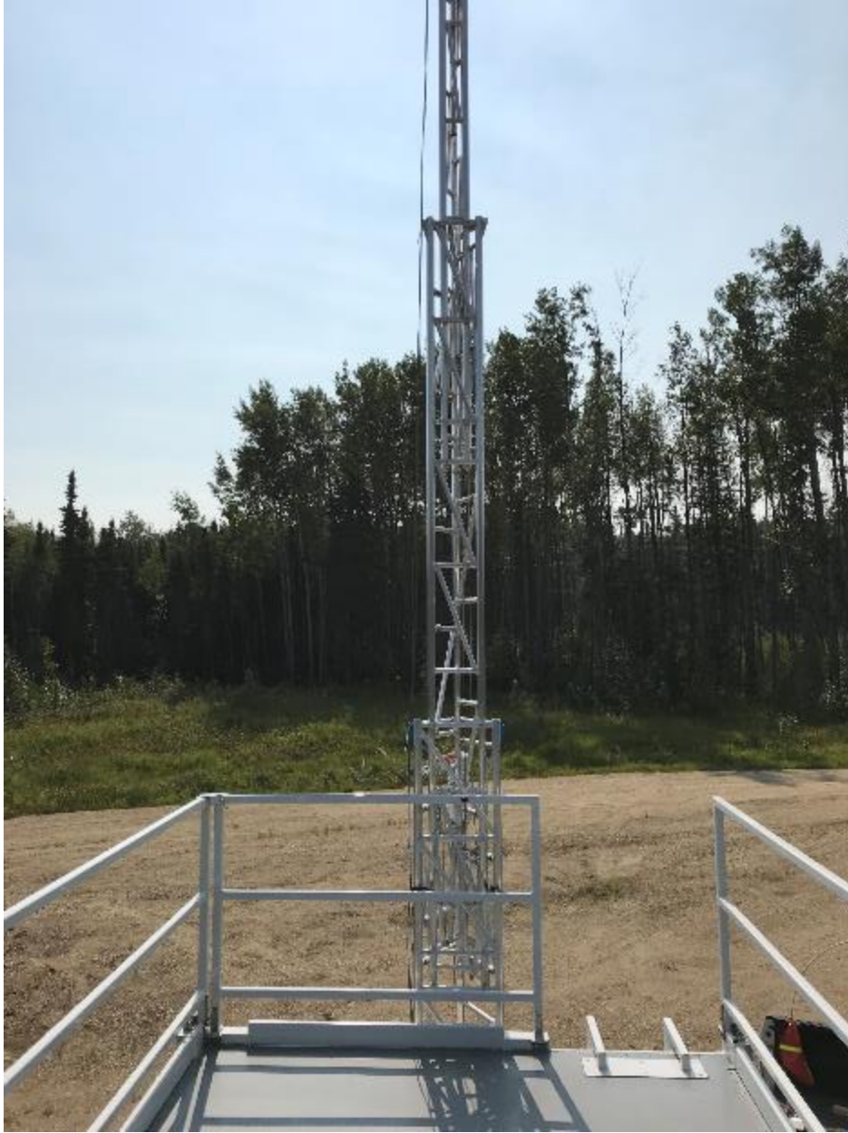
Figure 5.1 – Environ Looking East
