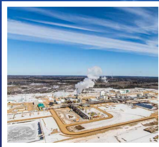
A SAGD facility in the southern Regional Municipality of Wood Buffalo.
